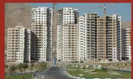
Rojan Building mass- Tehran
