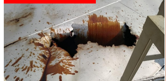
Fig. 3: Hole in top of hot oil tank
