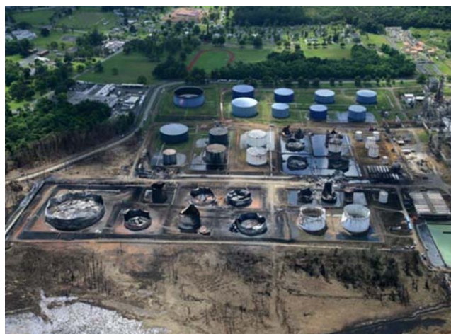
Damage to the facility after the fire
