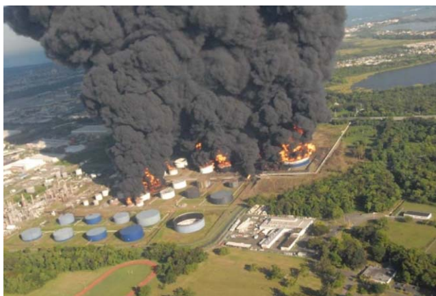
Multiple tanks burning in the fire
