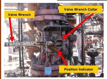
Many people would expect this valve to be closed - the position of the valve handle (in this case, a "valve wrench") is perpendicular to the pipe. But close inspection of the valve position indicator shows it is parallel to the pipe, clearly indicating the valve is open! WHY? The valve wrench collar is square and can be positioned in two ways — one with the valve wrench parallel to the valve position indicator and the other with the valve wrench perpendicular to the position indicator.
