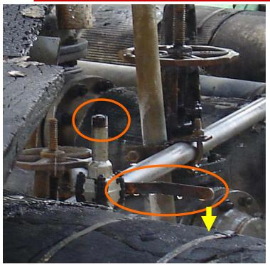
A piece of debris fell from temporary scaffolding used to support people and material. It fell onto the straight handle of a quarter turn ball valve on a ¾-inch (about 20 mm) vent on a large process pipe. The falling debris caused the vent valve to open. The large pipe contained flammable material, which was released through the vent. The released material ignited. The resulting fire killed one contract worker and seriously burned two others.
