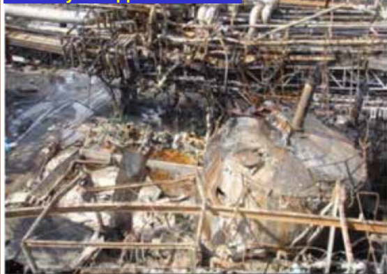
Photo 1: Destroyed AA Tank
