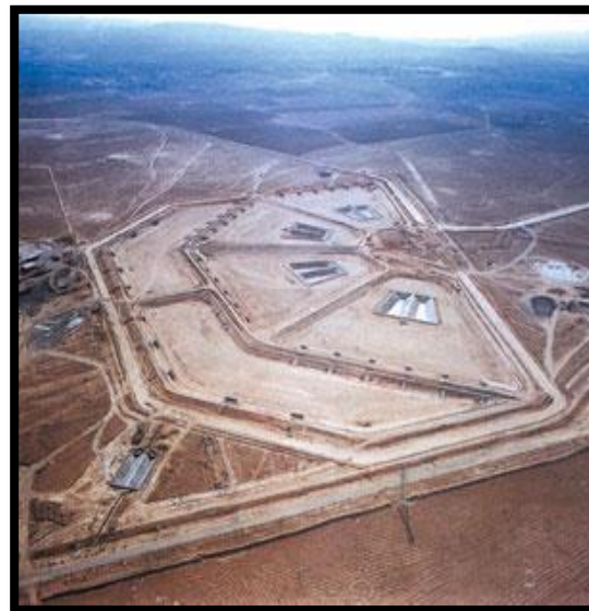
Fig.1: Overview of treatment plant
