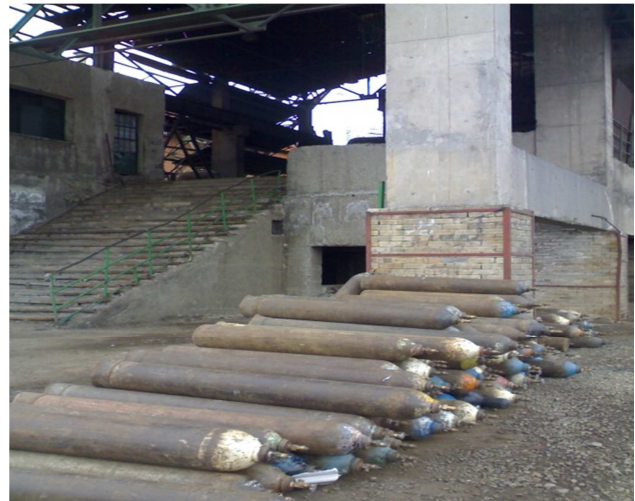
Figure 2. Oxygen cylinders position before the intervention
