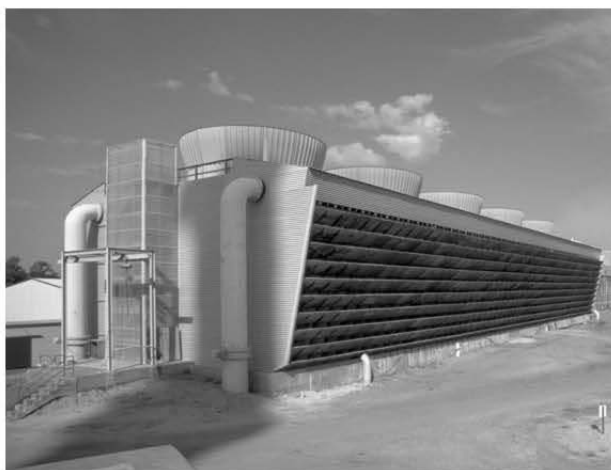
FIGURE B.1(e) Typical Induced-Draft Crossflow Water-Cooling Tower.
