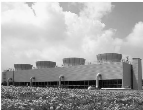
FIGURE B.1(d) Typical Induced-Draft Counterflow Water-Cooling Tower.
