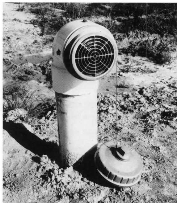
Figure B-5.1(a) Dry hydrant.
