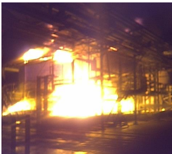
Figure 1. Tanks ablaze after a lightning strike
