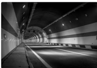
Road tunnels and access tunnels
